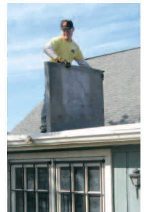
Jim Bochicchio removes debris from a roof. PHOTO BY LISA MULVEY
